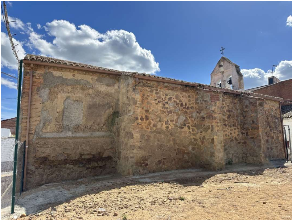
Side view showing the stone wall. © ARCHDIOCESE OF TOLEDO. TOLEDO. SPAIN
