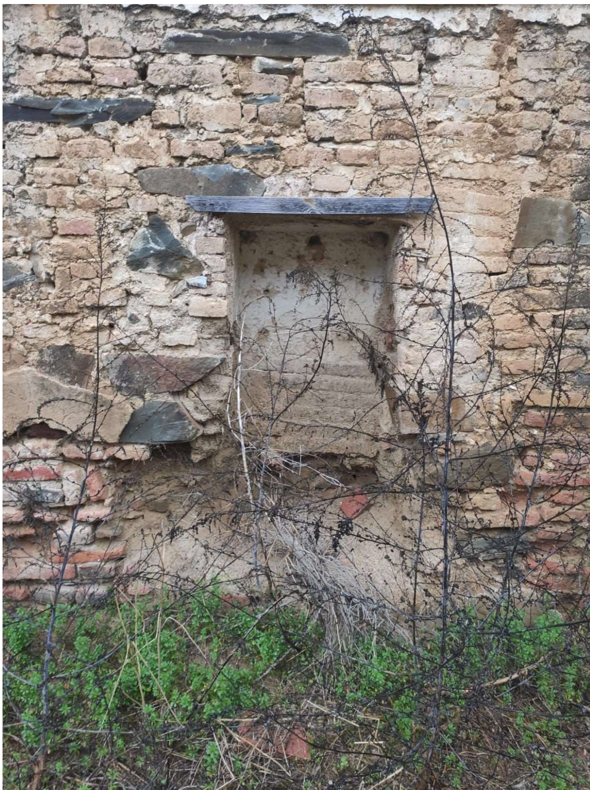
Blocked-up window in one of the walls of the former hermitage.
