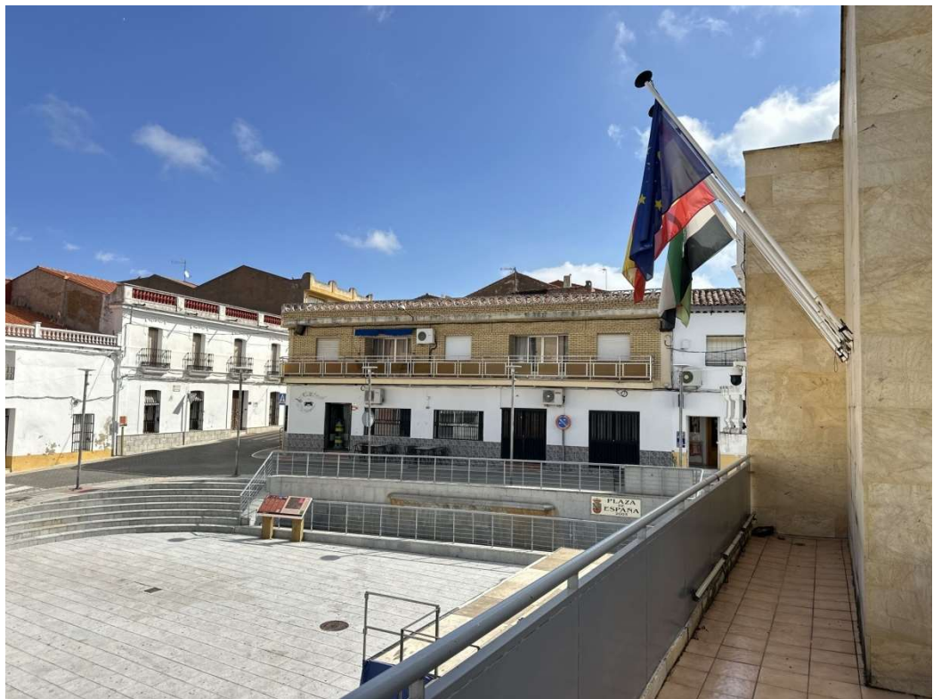
Images of the renovated Plaza de España viewed from the Town Hall.
