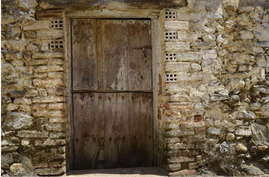
Detail of a wooden door in a house built with stone, adobe and brick in the Perchel neighbourhood.
