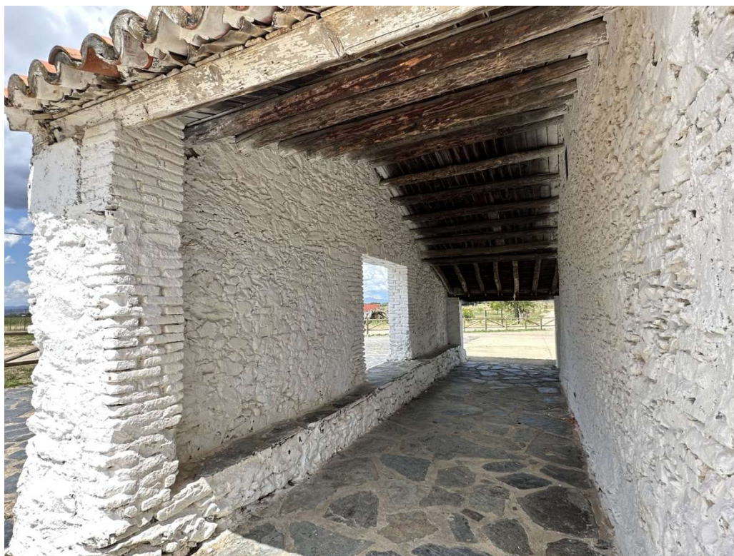
Portico supported by brick pillars.
