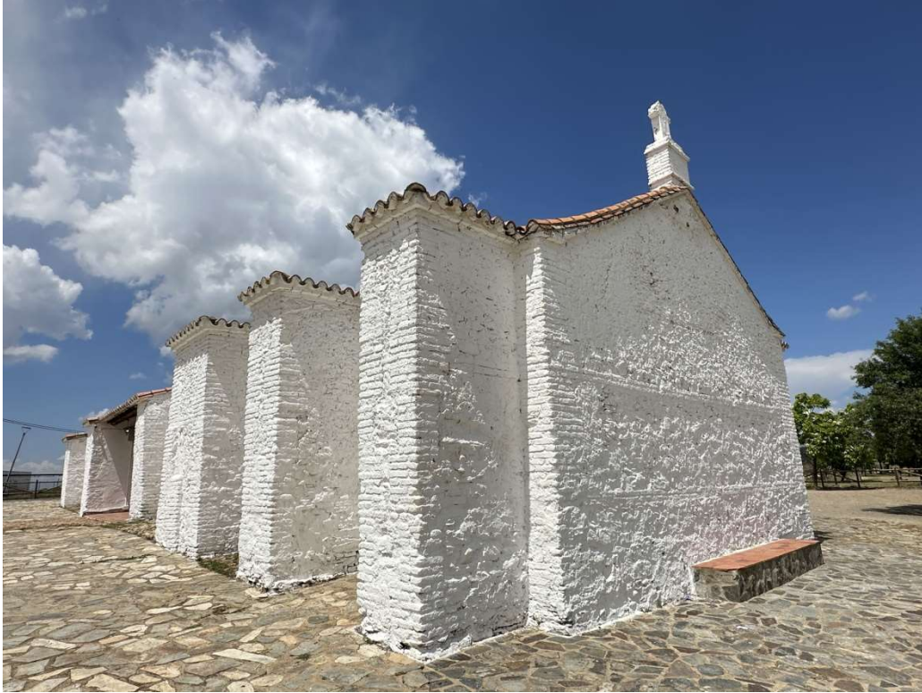
Buttresses on one side of the hermitage.
