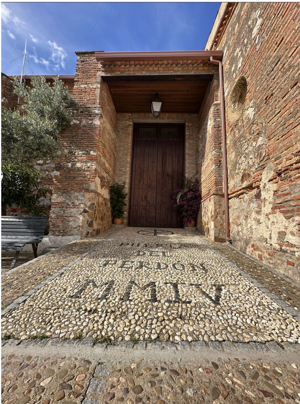
“Puerta del Perdón”, recently reopened and enlarged to improve accessibility.
