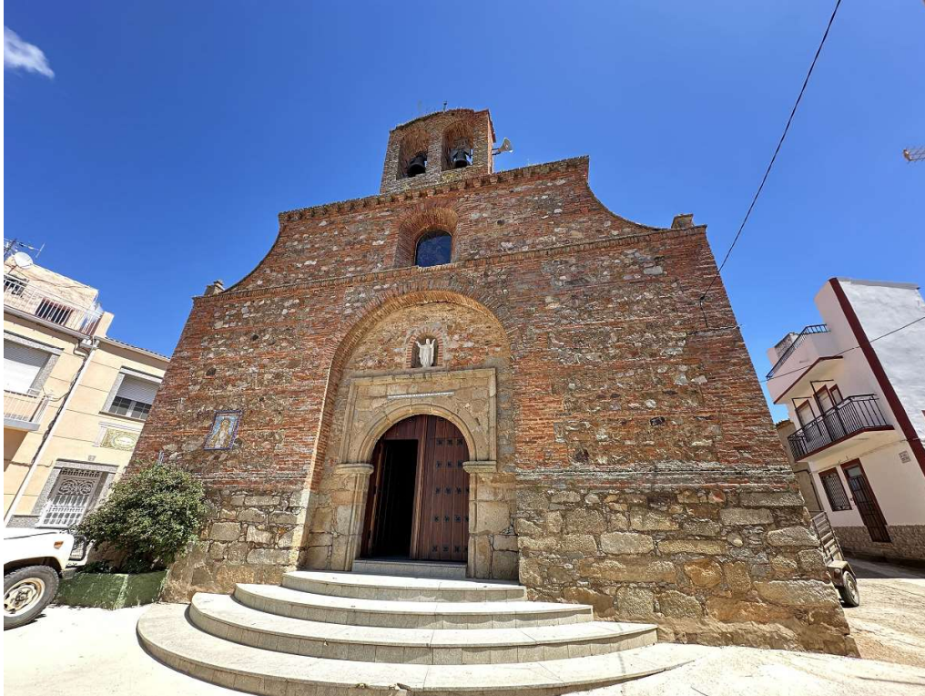
Front view of the single-nave building. © ARZOBISPADO DE TOLEDO. TOLEDO. ESPAÑA
