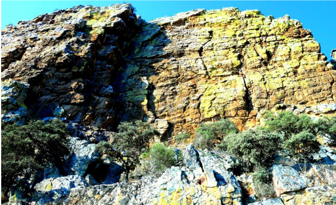
Vegetation, the isolation of the enclave, and the passage of time have contributed to its deterioration. FOTOS: JOSÉ ANTONIO BERMEJO.
