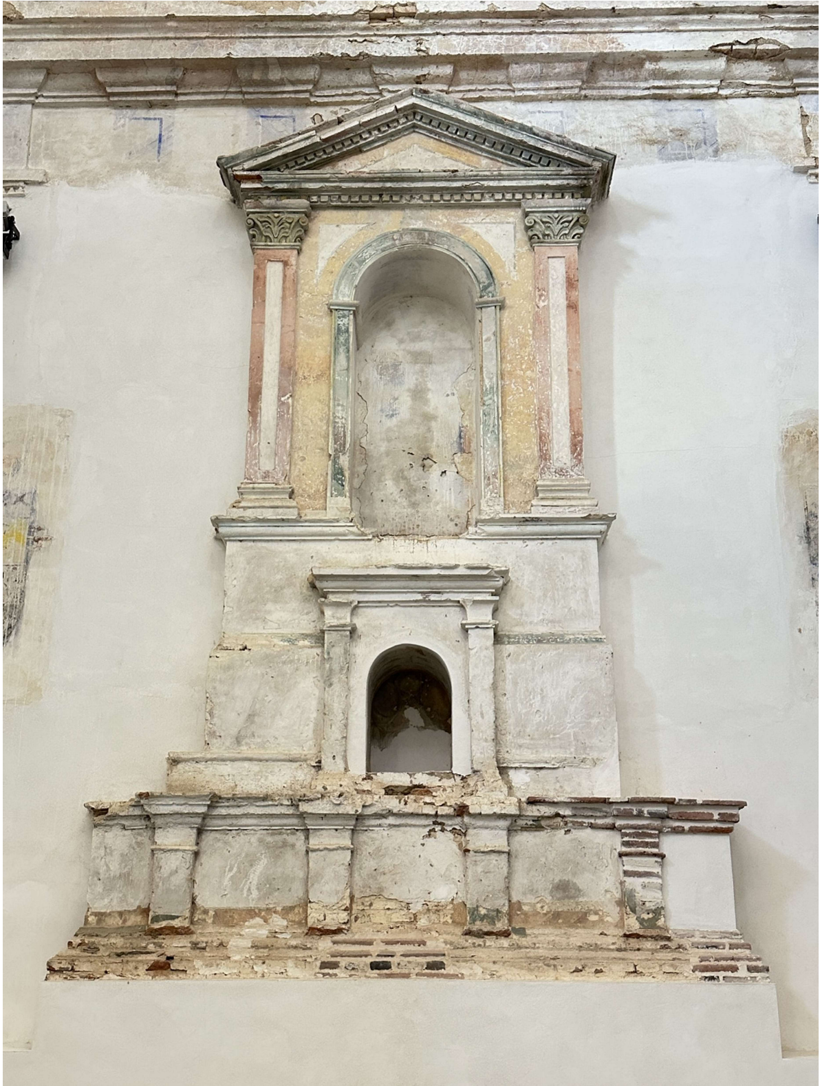
The cloister was formed by semicircular arches, partially preserved today.
