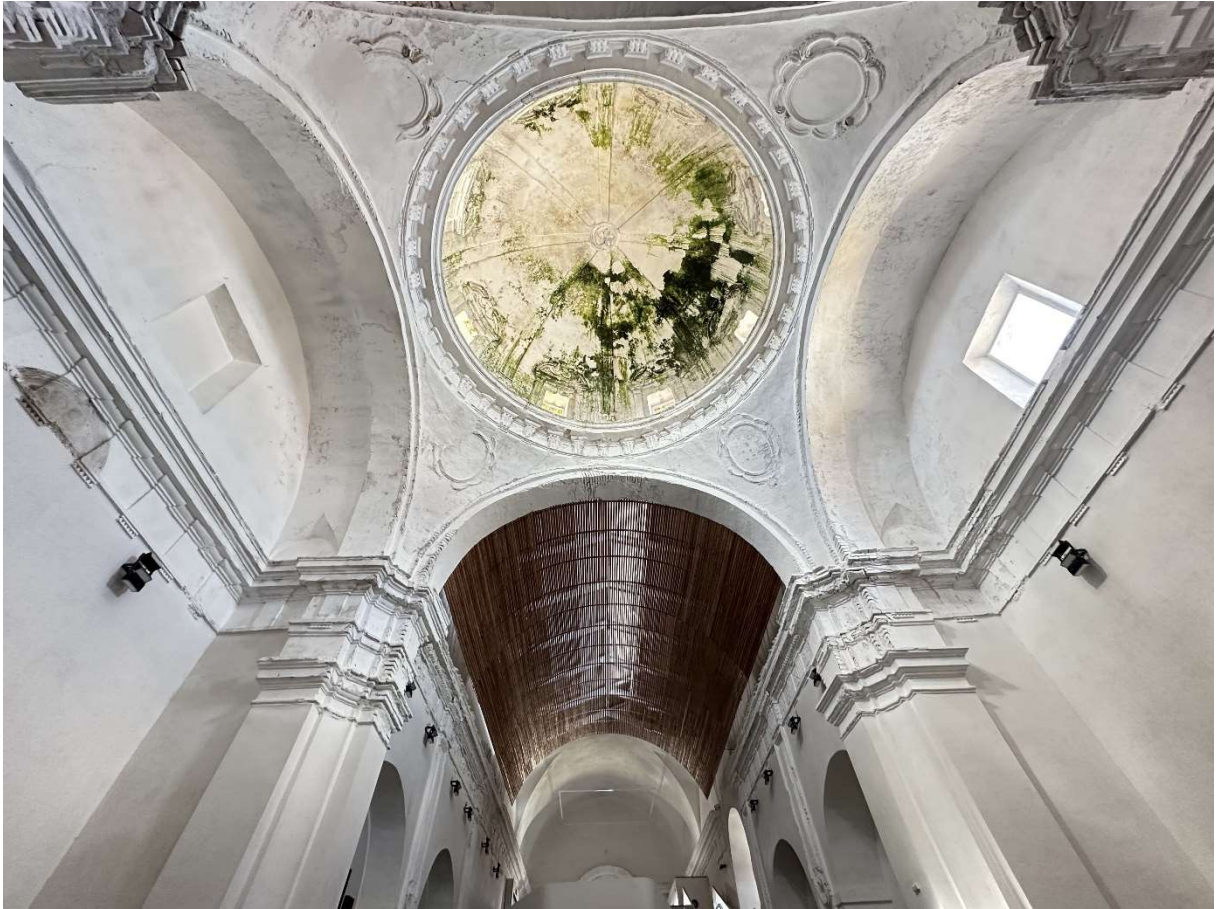
Current condition of the dome.
