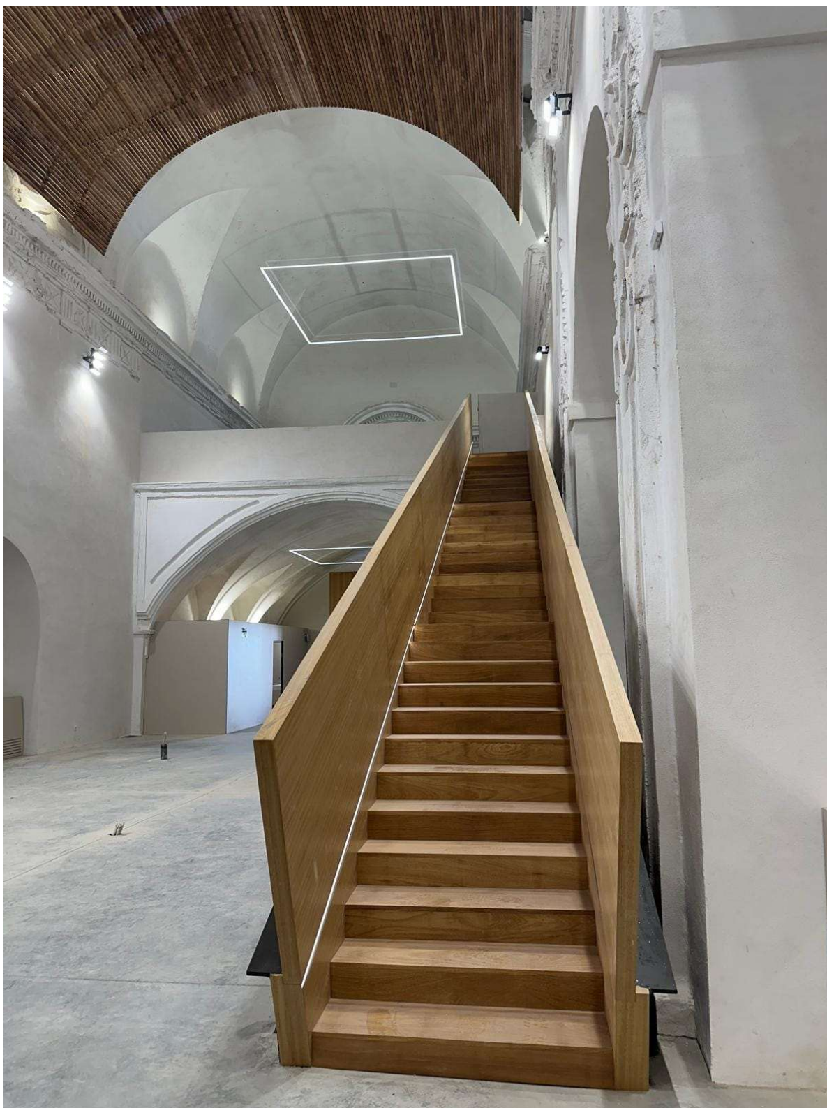
Interior view of the building after completion of the restoration process.
