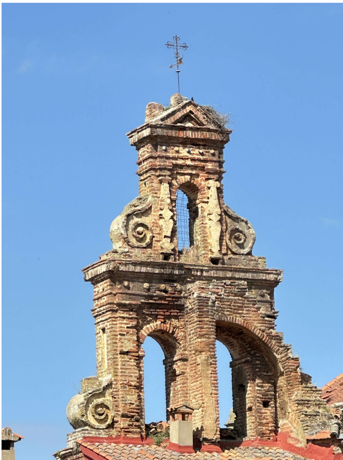
Bell gable of the convent without bells.
