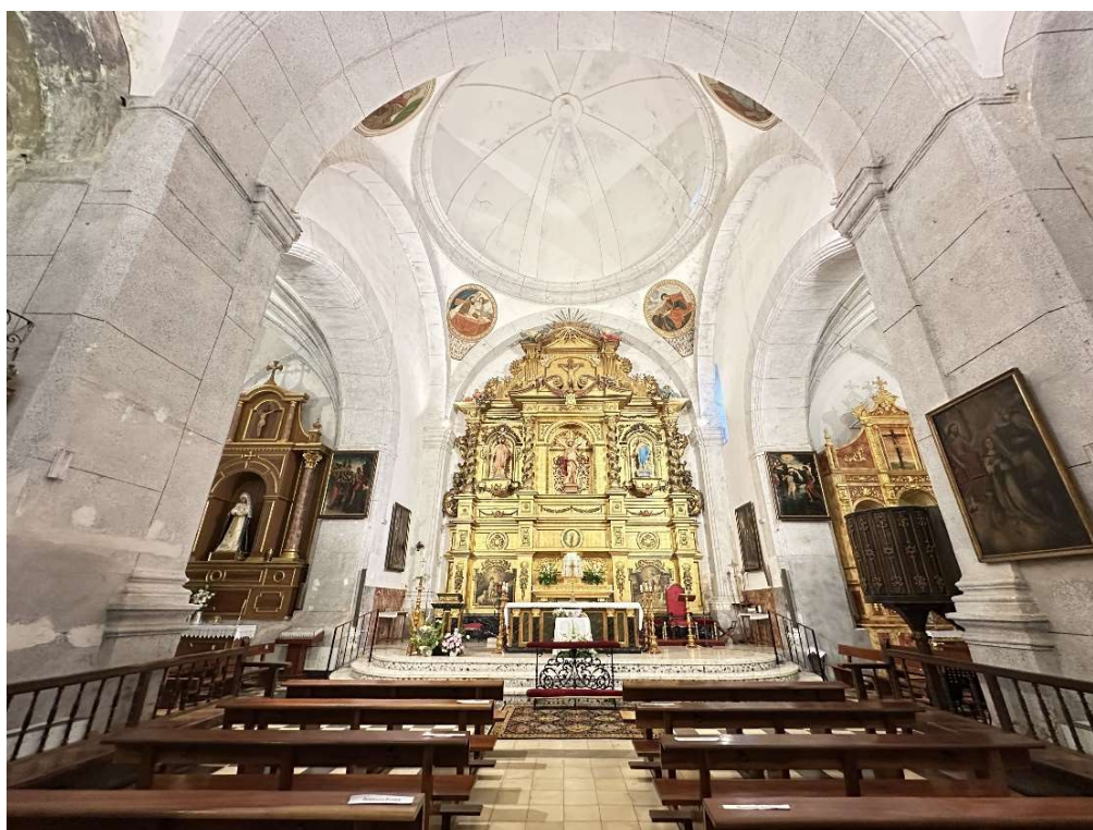
Different construction phases and stylistic contributions can clearly be identified within the church. © ARZOBISPADO DE
