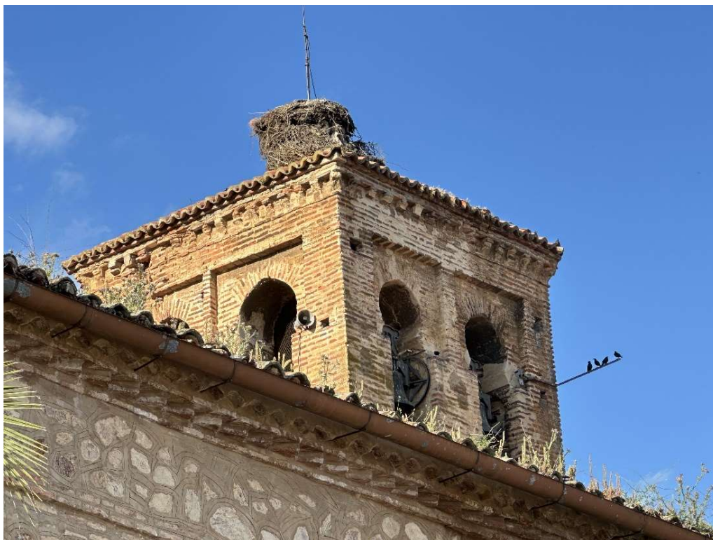
Powerful bell tower standing out prominently from the church.
