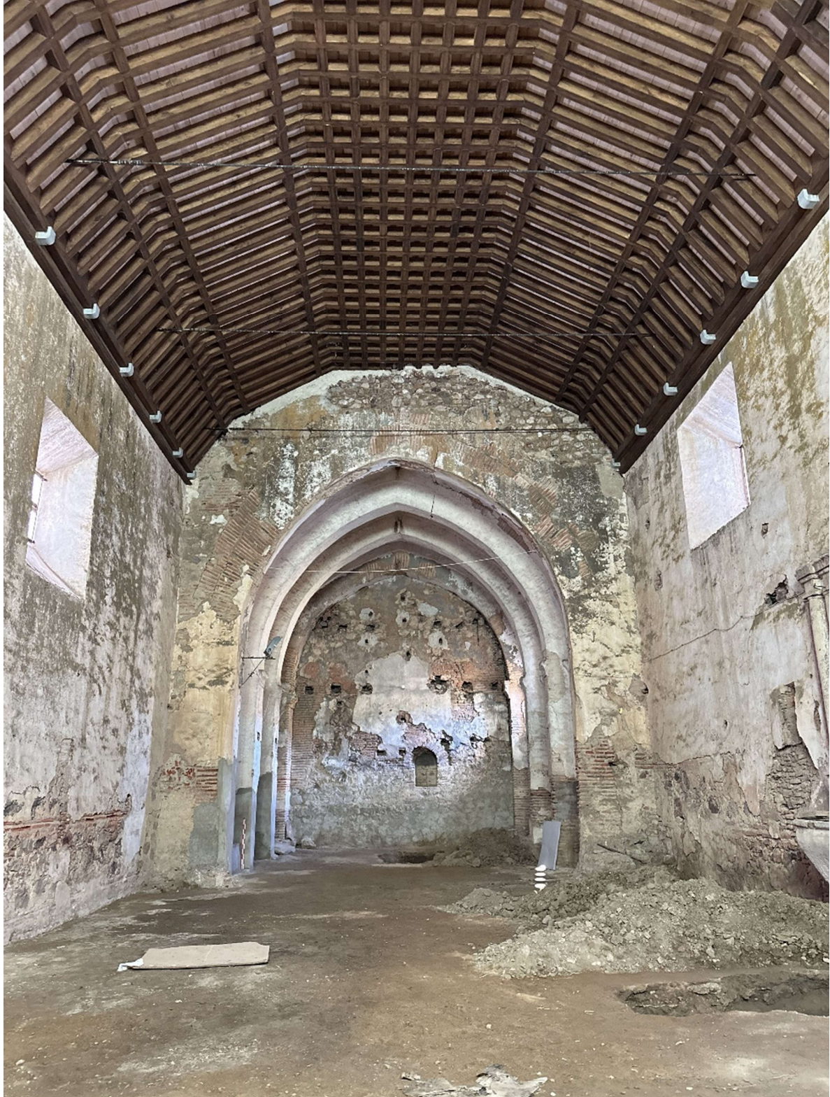
Convent church, where the wooden ceiling can be seen.
