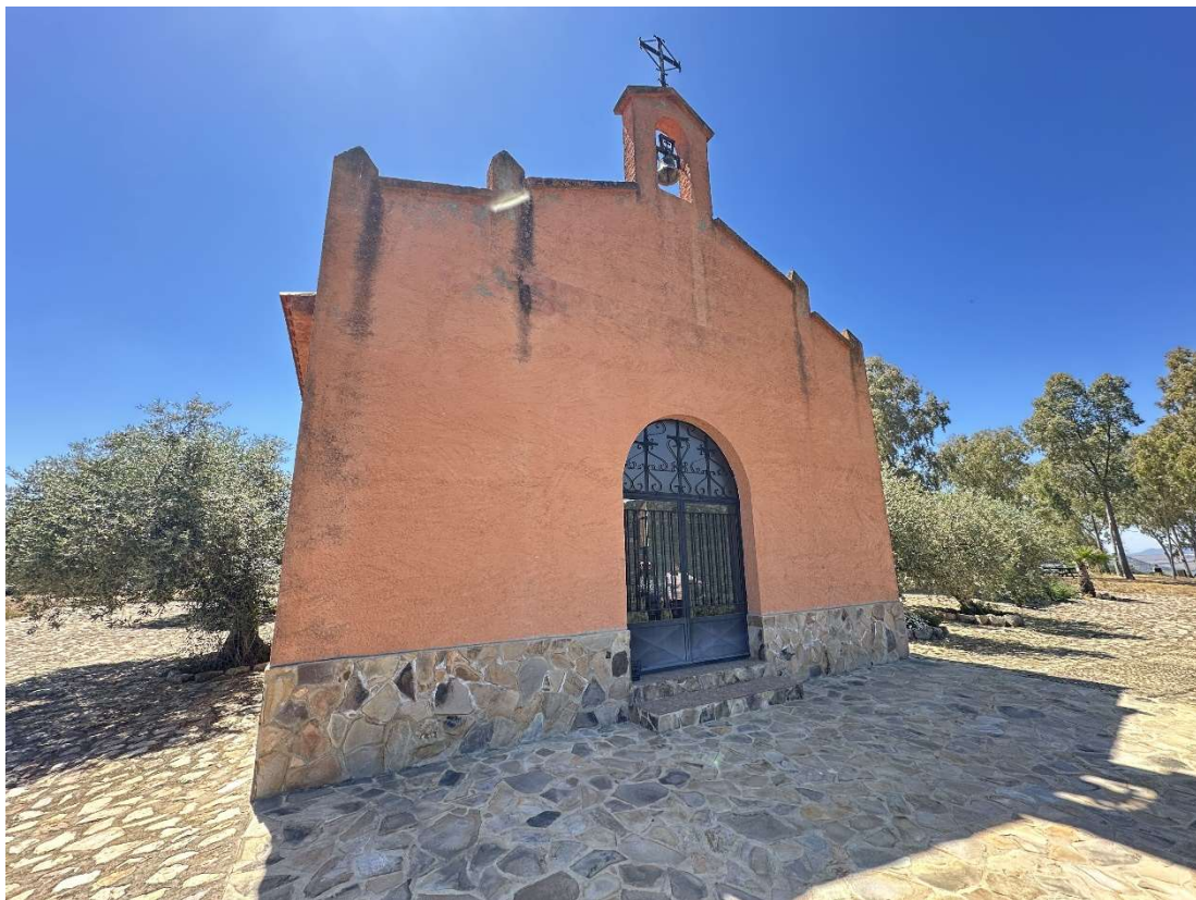
View of the hermitage, located beside an olive grove. © ARZOBISPADO DE TOLEDO. TOLEDO. ESPAÑA
