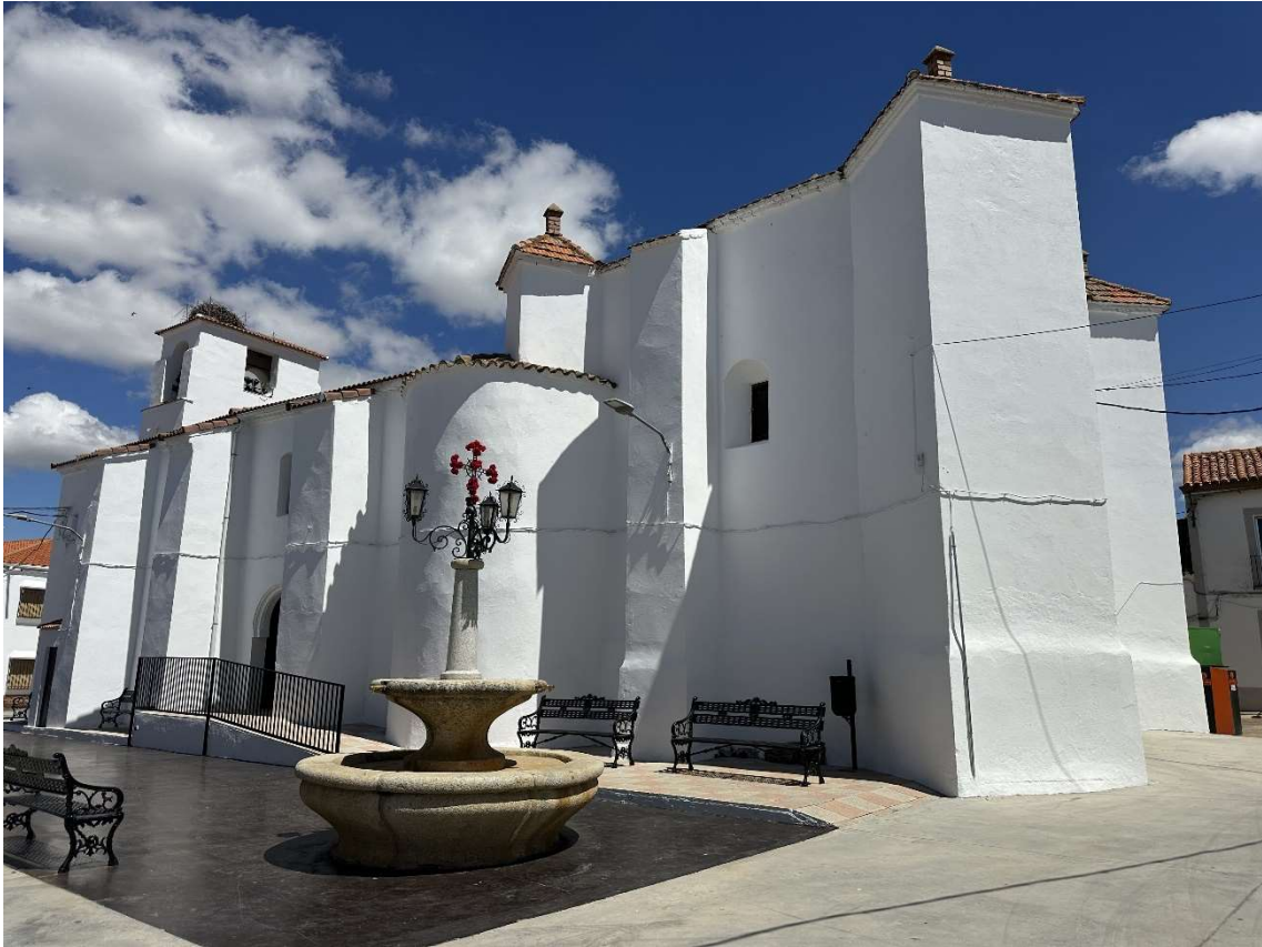
Lateral buttresses of the nave, crowned with restored brick pinnacles.
