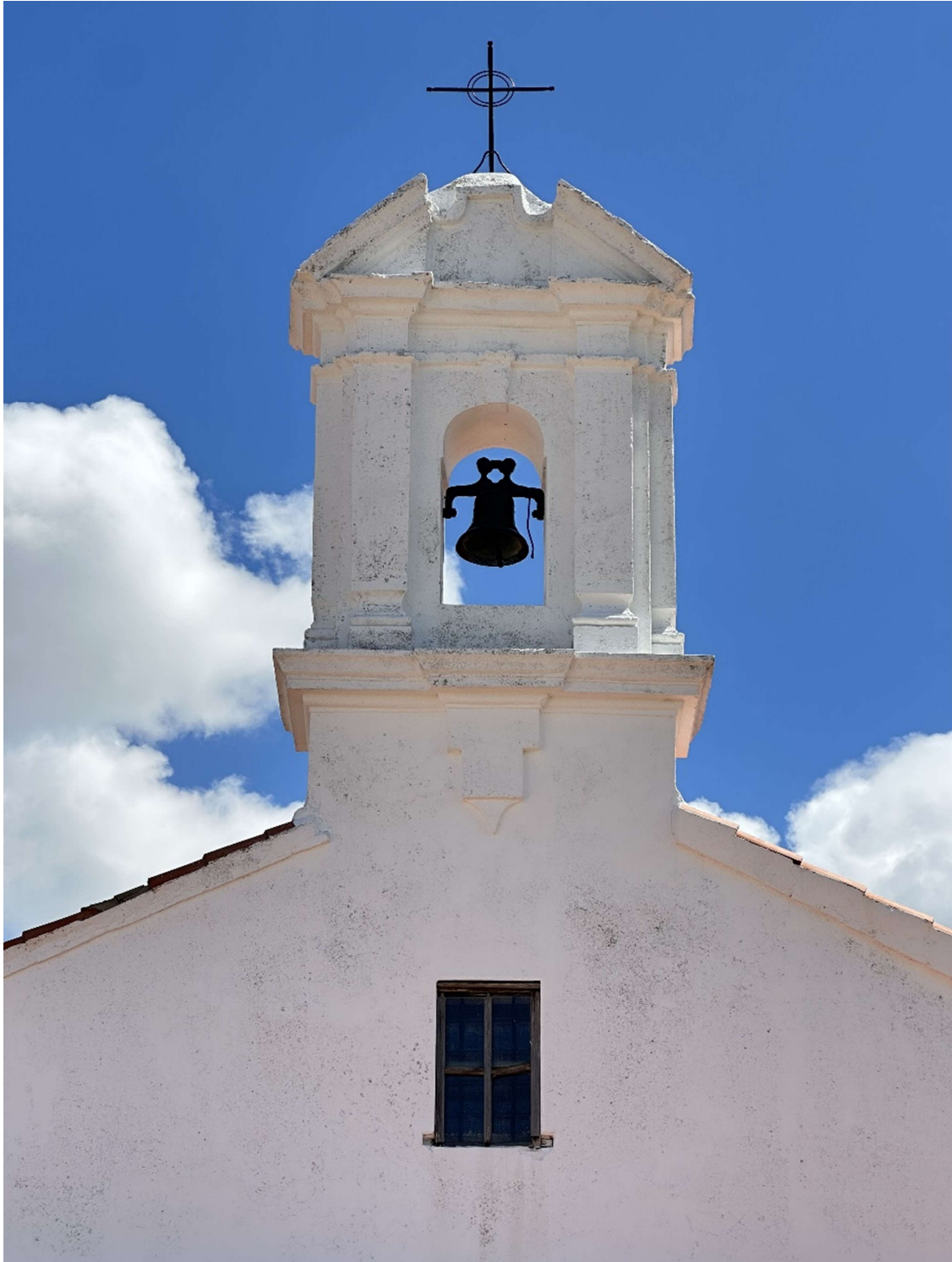
Bell gable with a bell topped by a cross at the upper part. © ARZOBISPADO DE TOLEDO. TOLEDO. ESPAÑA
