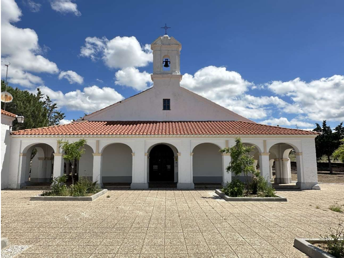
View of the main façade of the hermitage, with a porticoed area of seven arches.
