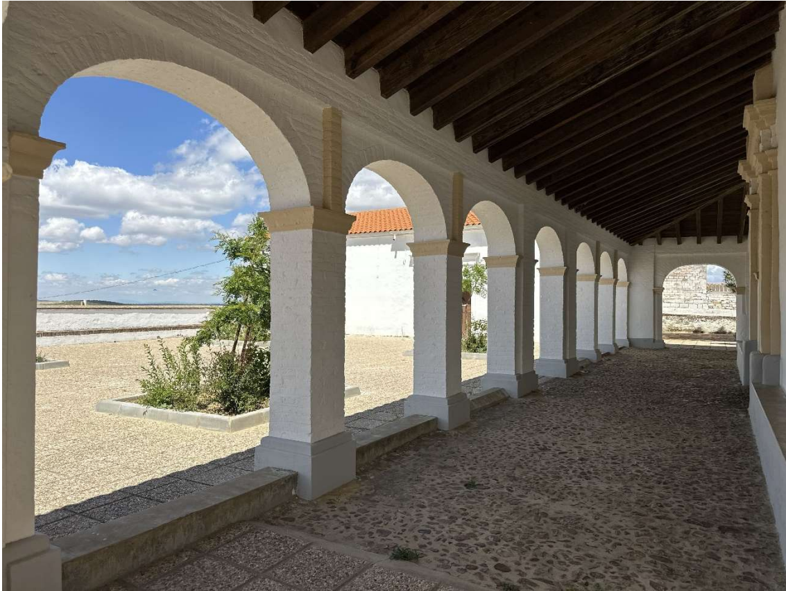
Porticoed area of the hermitage at the entrance. © ARZOBISPADO DE TOLEDO. TOLEDO. ESPAÑA
