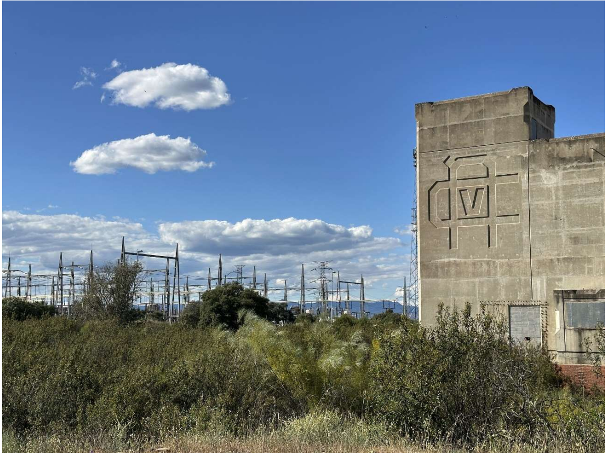
Image of the building intended to house Unit II. In the background, the electrical substation supplying the municipality.
