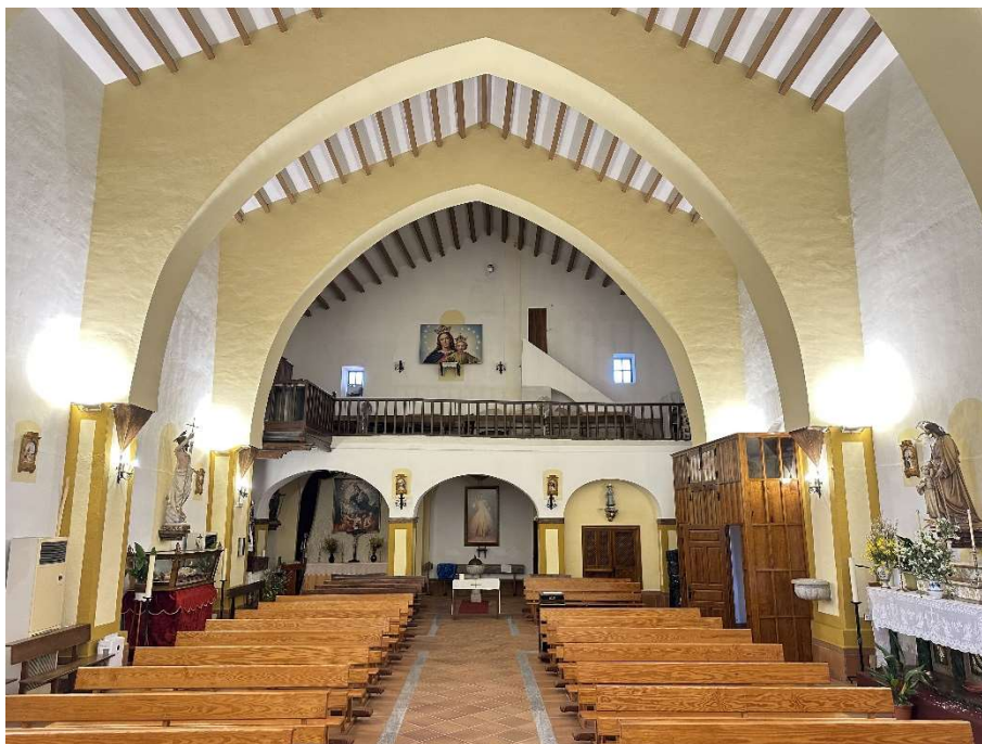
The church has a three-nave floor plan separated by diaphragm arches and gabled roofs. © ARZOBISPADO DE TOLEDO. TOLEDO. ESPAÑA
